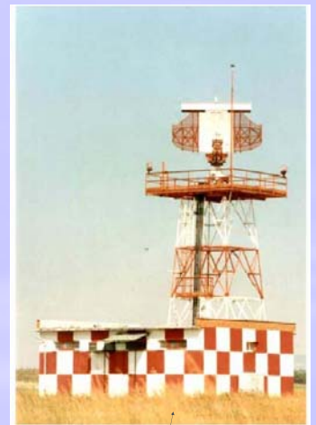
ATCR-33K without radome. ASTERIX CAT 8 weather contours
