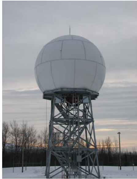
(Left) The new 3-meter X-Band satellite receiver dish at Elmendorf Air Force Base, Alaska, shielded from the elements by its protective dome. (Right) MARK IVB, Terra satellite imagery with snow-land multi-spectral imagery algorithm.
